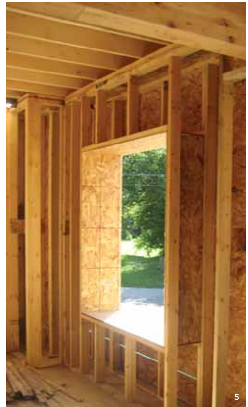
AS WITH ALL EQUILIBRIUM HOUSES, THE RIVERDALE PROJECT IN EDMONTON HAS A HIGHLY INSULATED ENVELOPE, IN THIS CASE ACHIEVED WITH A DOUBLE WALL CONSTRUCTION THAT, ACCORDING TO THE BUILDER, HAS LOW INCREMENTAL COST. [5] [Photo Habitat Studios]
